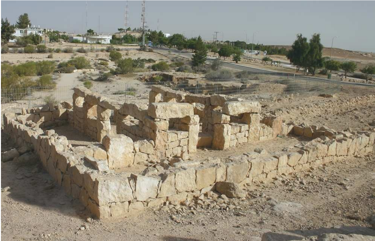
Rebuilt four-room house. A typical Israelite dwelling down to the Babylonian exile (586 BC). Three parallel rooms and one long cross room.
