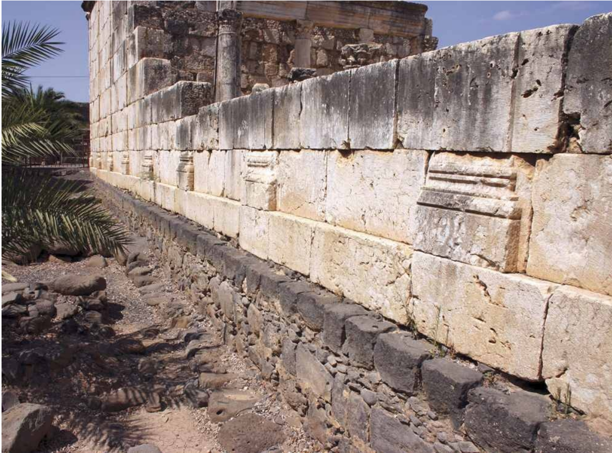
Black basalt foundation wall of an earlier synagogue upon which the rebuilt white walls of the sixth-century synagogue at Capernaum are visible
